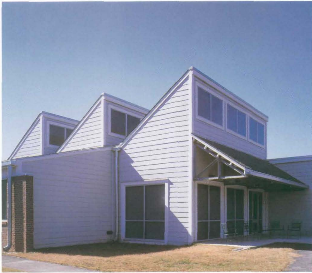
(top) The jagged roofline and choice of materials differentiates the cottages from the older buildings and create a sense of community; photo by Hester + Hardaway. (bottom) Because of the overhead lighting, even areas with no exterior windows seem light and airy; photo by Taft Architects.
