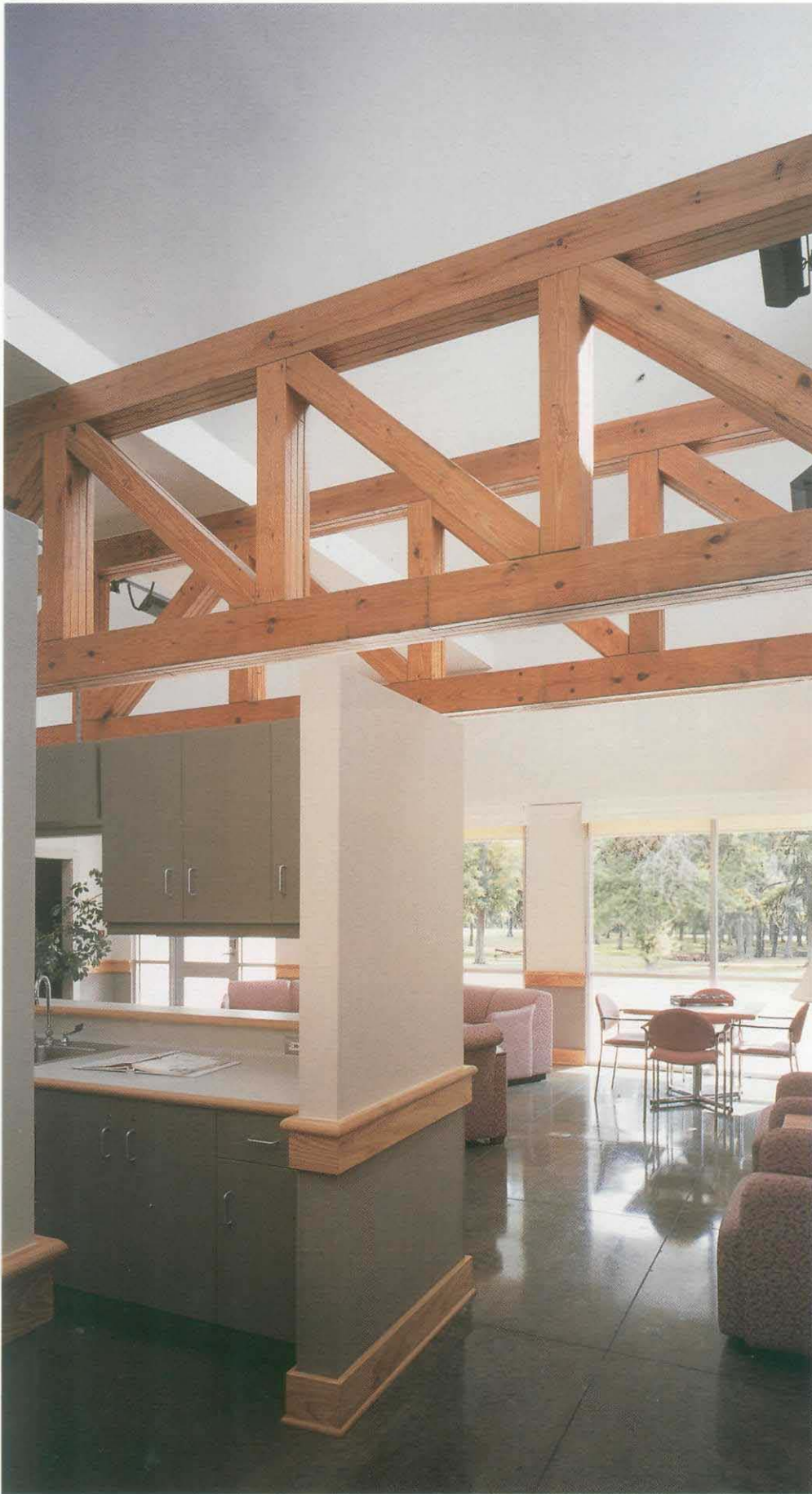
(opposite page) Auto traffic is relegated to the outside edge of the complex, providing the cottages with a quiet communal backyard; photo by Taft Architects. (this page) Large gang-nailed trusses support north-facing skylights; photo by Hester and Hardaway.
